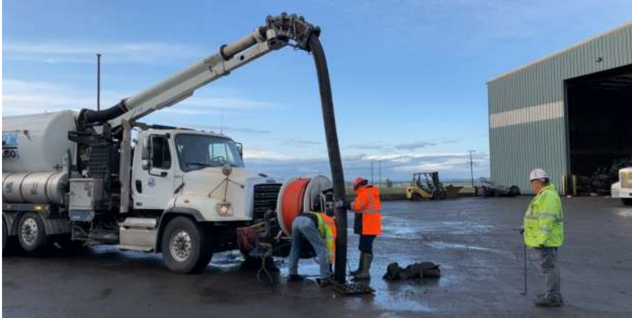
Figure 11-1. A County crew cleans out a catch basin at the Skagit County Transfer Station.
